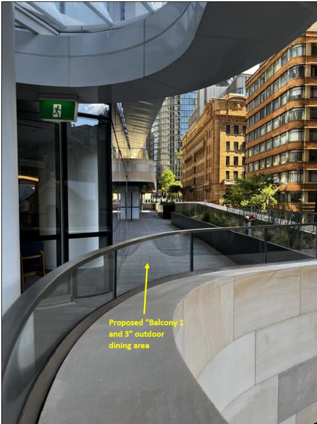
Figure 6: Southern-most section of outdoor seating (identified as Balcony 1 and 3 on the plans)
